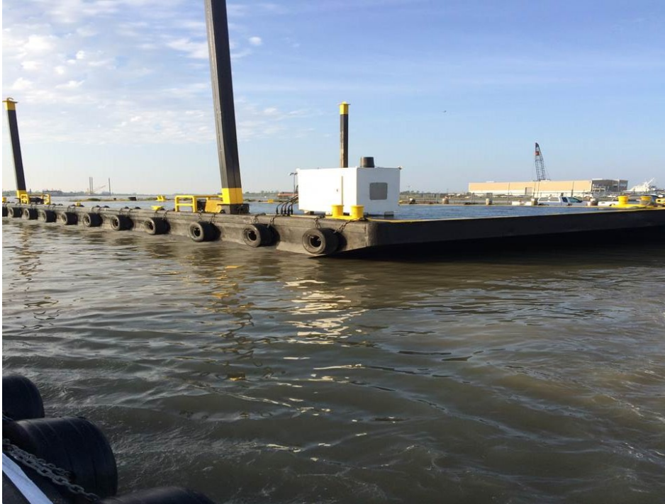
Diesel pulling unit (2) 35'x16" Square Spuds
